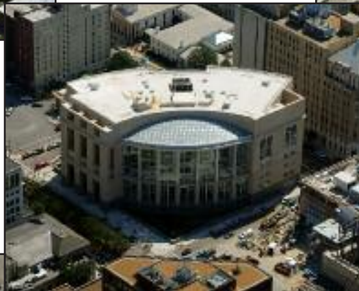
Richmond Federal Courthouse
