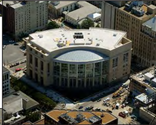
Richmond Federal Courthouse
